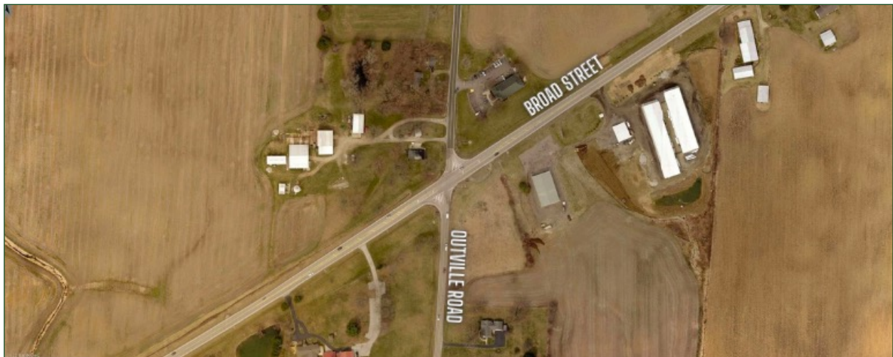
IMAGE 4: Outville Road at Broad Street
