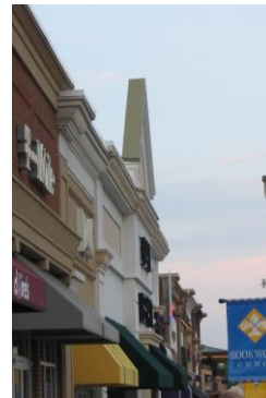
Figure 26.04: The image on the left illustrates the use of parapet walls to screen mechanical equipment. Tall, thin parapets such as the one shown in the image on the right should be avoided to prevent the appearance of false walls.
