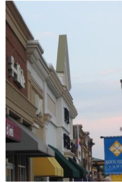
Figure 26.06: The image on the left illustrates the use of parapet walls to screen mechanical equipment. Tall, thin parapets such as the one shown in the image on the right should be avoided to prevent the appearance of false walls.
